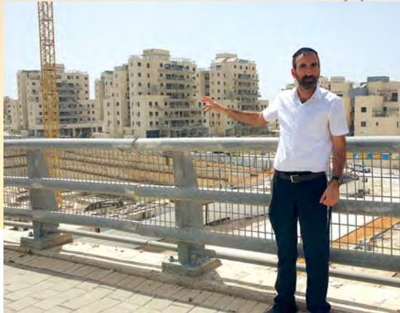
Benzi Rakov leading a tour of a residential construction project for the haredi community
